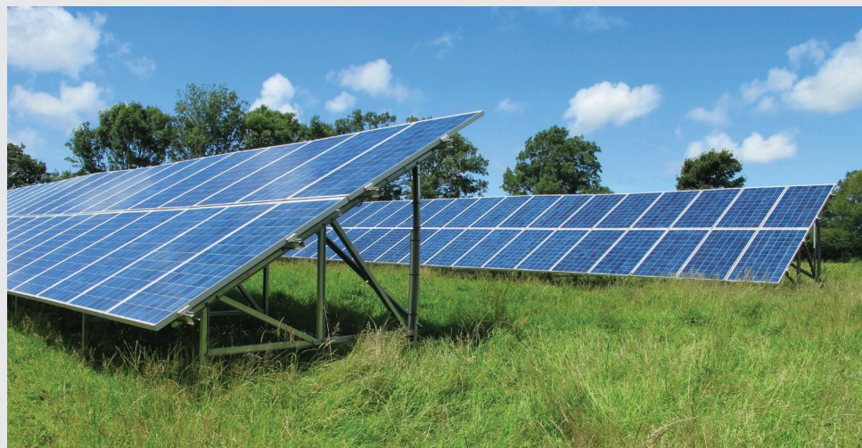
Lightsource has developed a bespoke SCADA system for its growing fleet of PV plants.
