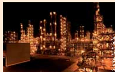
LDK Solar's TCS plant. Metallurgical silicon is used as a raw material to produce TCS, which is then used to produce polysilicon.
