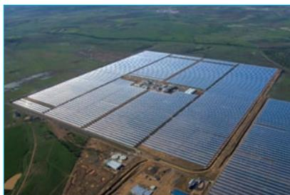
GE Energy Financial Services is investing with German fund KGAL in a 50MW parabolic trough concentrated solar power plant using molten salt energy storage, shown here, in Badajoz, Spain.
