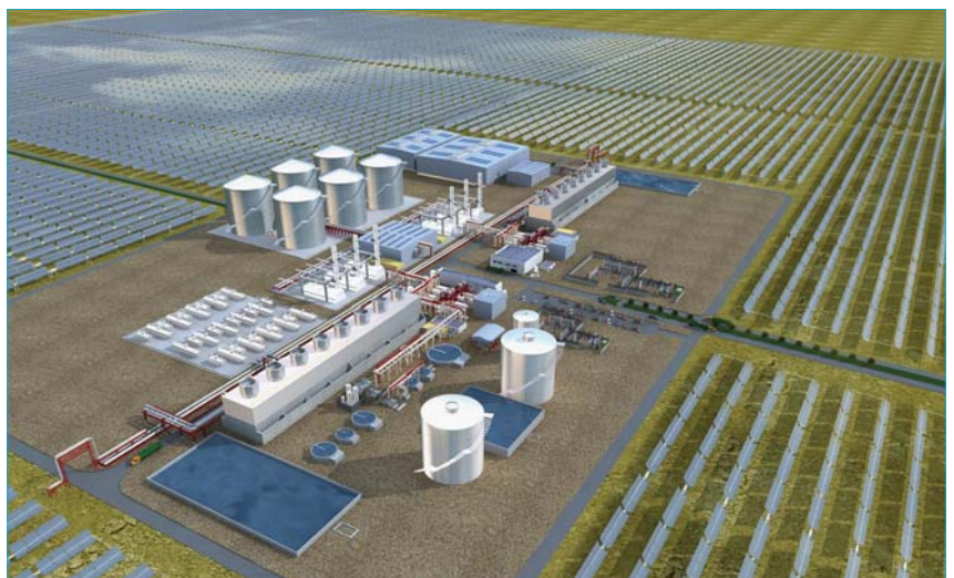
Abengoa Solar uses parabolic trough technology
