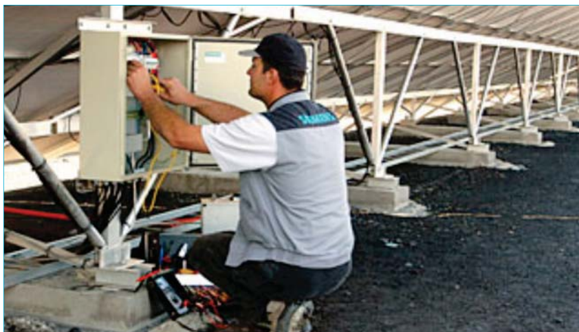
Figure 1. A Siemens engineer installing modules at a City Solar facility.
