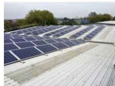
Upstanding South Facing system on East/West pitches
