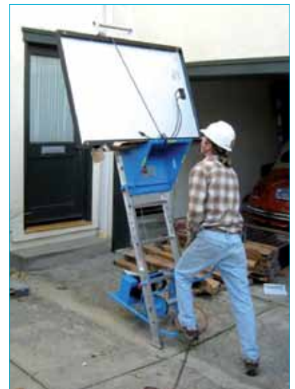
Figure 3. Specialized module lift mechanism.
