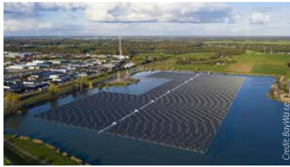
The recently completed 14.5MWp Sekdoorn plant in the Netherlands was designed to optimise the levelised cost of electricity, according to developer Baywa r.e.
