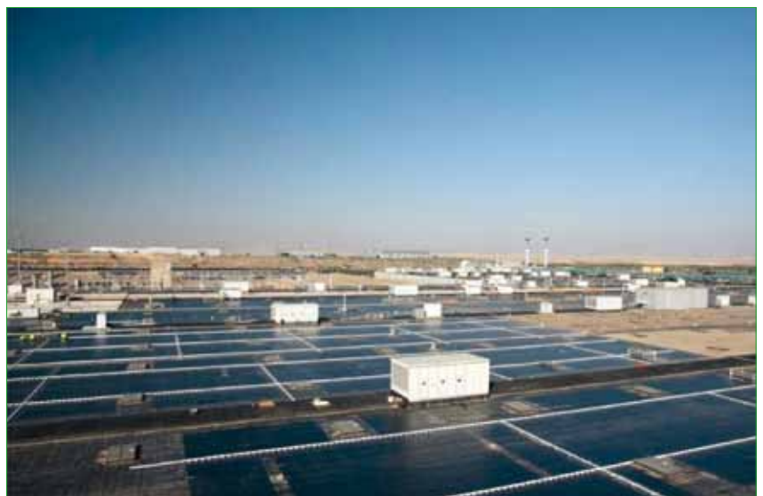
Figure 1. World's largest rooftop system (11.8MW) in Zaragoza, Spain. The system uses flexible thin-film silicon PV laminates.
