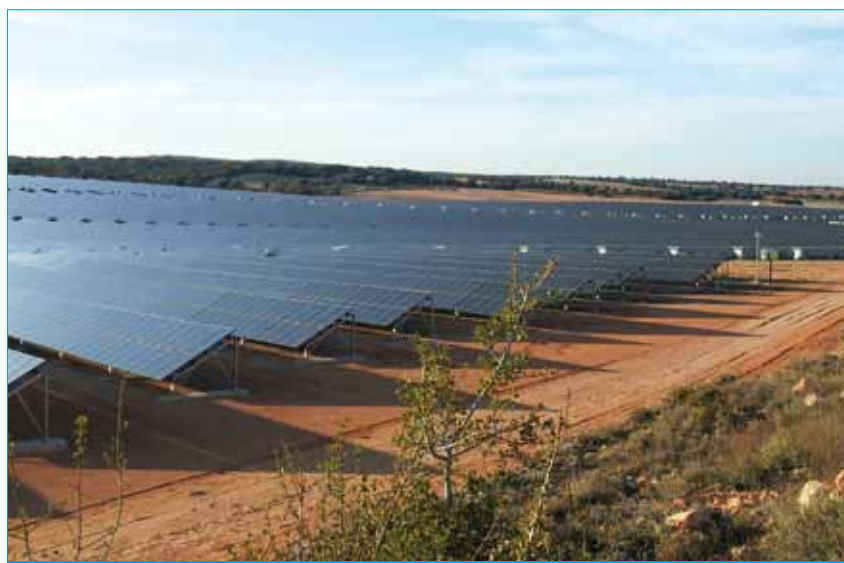
Figure 1. View of a 10MW utility-scale PV installation in Osa de la Vega, Spain.
