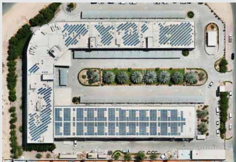
Distributed solar in the MENA region has had some success, such as in Dubai, but been constrained by the low cost of power for C&I customers
