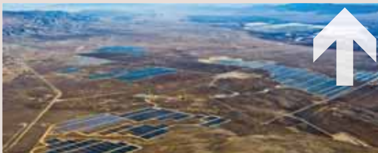
Source: SunPower Corporation
