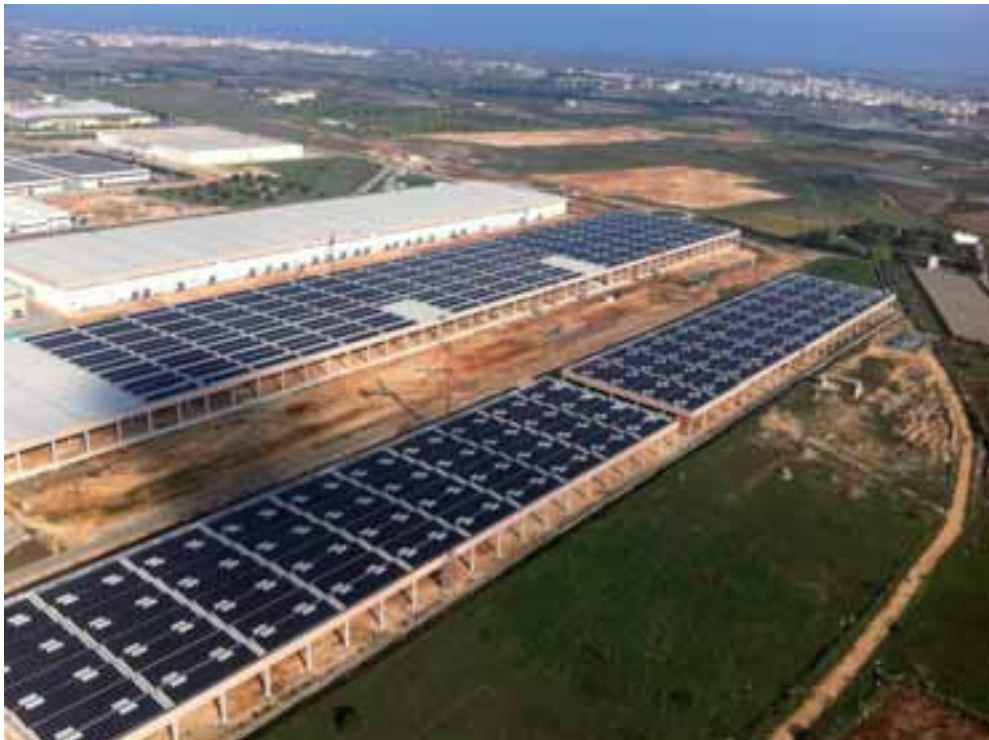
A 3.1MW on-site bonded project in Bari, one of Italy's largest PV installations.
