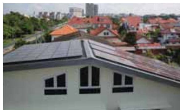
Figure 6. The first zero-energy house in Singapore: the east-facing roof is tilted at 18.3° (right side of the roof), while the west-facing roof is tilted at 6.1° (left side of the roof).
