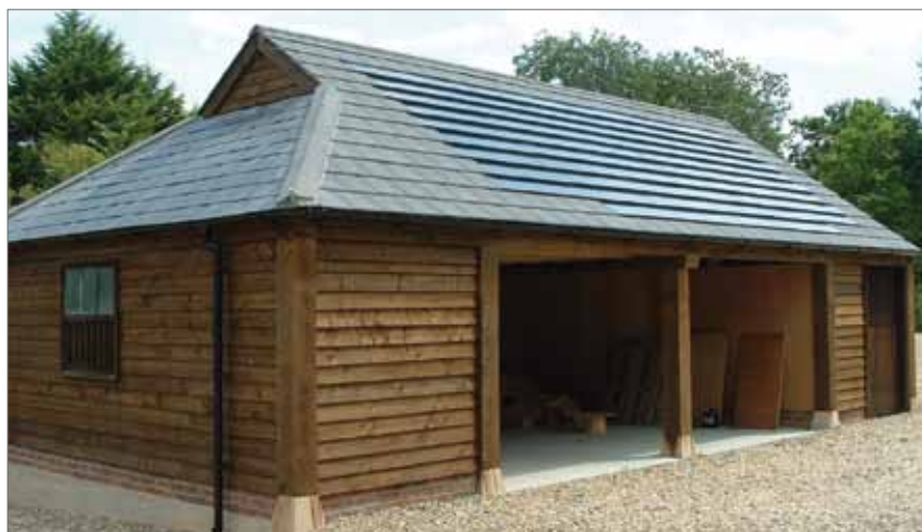
Figure 2. C21e solar electric roof tiles on a building in Sturges Farm, southwest England.
