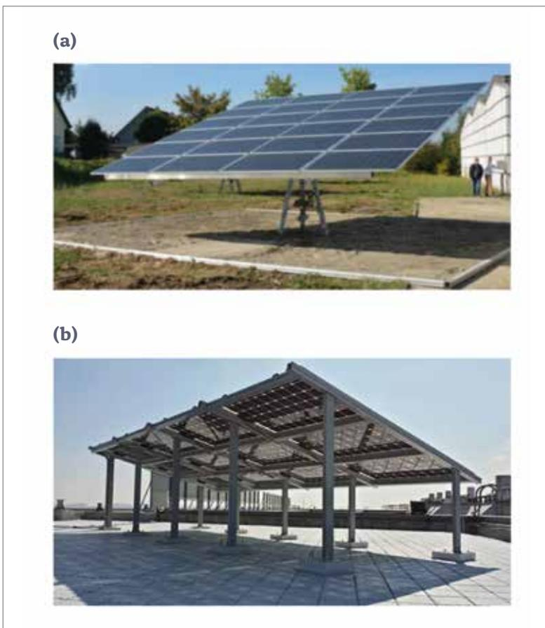
**Figure 4. Field installations of bifacial modules using PERC+ solar cells: (a) 13kWp Bisun modules from SolarWorld mounted on a single-axis tracker system [27]; (b) 2MWp rooftop installation currently under construction by Neo Solar Power, implementing their Glory BiFi modules [29].**
