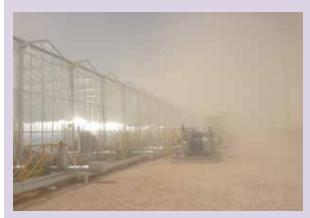
GlassPoint Solar last year secured a US\$53million in financing for an enhanced oil recovery (EOR) project. EOR uses steam to increase the return from the well. Remote oilfield operations usually use gas to generate steam. GlassPoint encloses a parabolic CSP system – inside a glass house to reduce the impact of dust - to generate the steam required.
