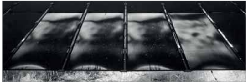
Figure 7. EL pictures taken on-site.
