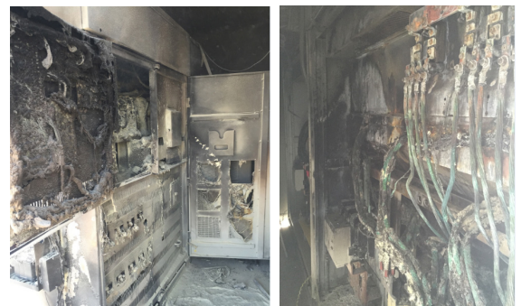
IGBT inverter explosion/fire hazard caused by poor inverter quality and technical design.
