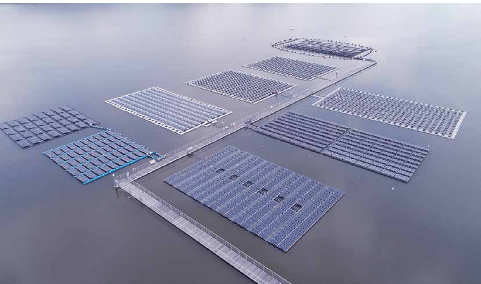
Figure 1. Singapore testbed of 10 different floating solar technologies on Tengeh reservoir
