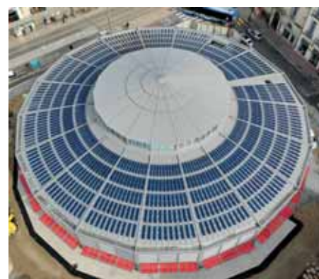
▲ The glass/glass modules are 50% transparent to allow visibility, according to the architect's specifications, of the grey metallic colour of the underneath roof cover
