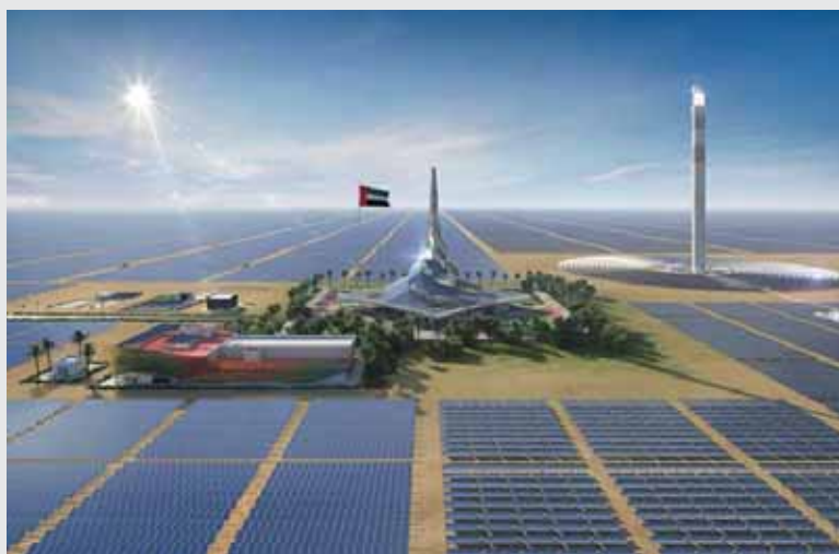
The 5GW Mohammed bin Rashid solar park.
