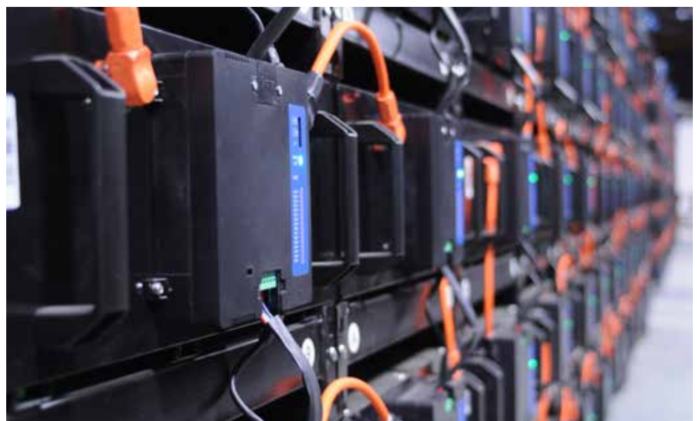
Credit: Powin Energy
