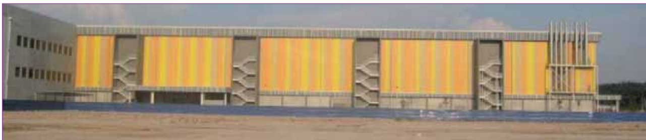
Figure 13. Side view of the Q-Cells cell manufacturing building in Malaysia.
