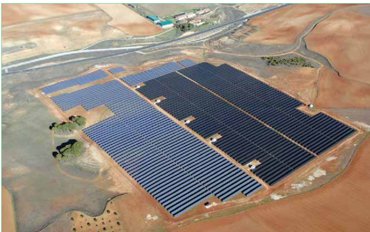
Figure 2. The Villanueva de la Jara PV power plant, Cuenca, Spain, consists of c-Si and CdTe modules, constructed by Phoenix Solar in 2008.
