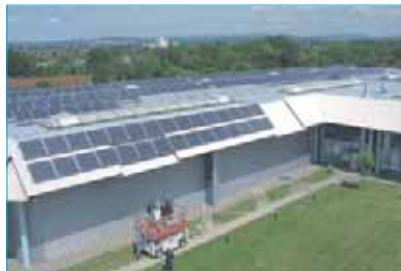
Figure 1. Industrial site of Hübner GmbH in Kassel (courtesy of ISET).
