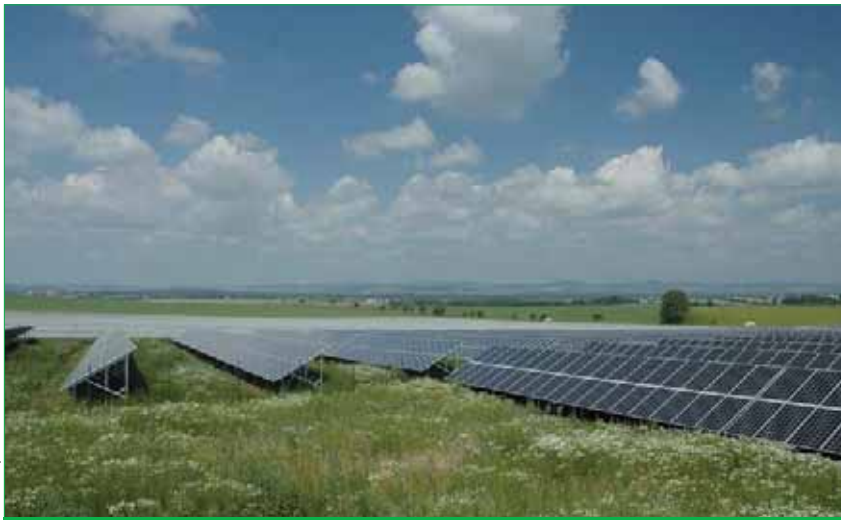
Figure 4. Ostrožská Lhota PV power plant was constructed in 2008 using c-Si modules. Ostrožská Lhota is one of the largest PV power plants in the Czech Republic, a country that has seen huge growth in recent months [4].
