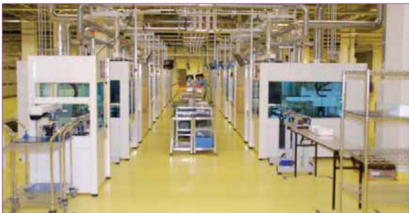
Figure 14. Overhead utility connections to process equipment in the manufacturing area.
