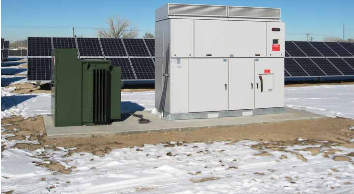
Figure 3. 500kW ground-mount PV system utilising a central architecture design; installed at the City of Greeley Water Pollution Control Facility.
