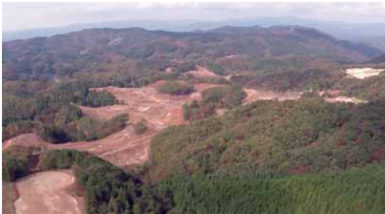
◀ Figure 5. Aerial perspective showing typical inhomogeneous topography, taken via drone during construction monitoring of a golf course being prepared for a PV power plant. Many PV projects are being developed in Japan at decommissioned golf courses, which were developed during the 1980s but later proved to be unprofitable. They have found a second life through PV plant development.
