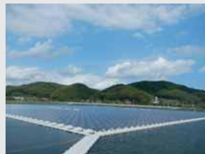
Floating PV plants, such as this one built by Kyocera, are seen as a solution to land shortages in Japan.
