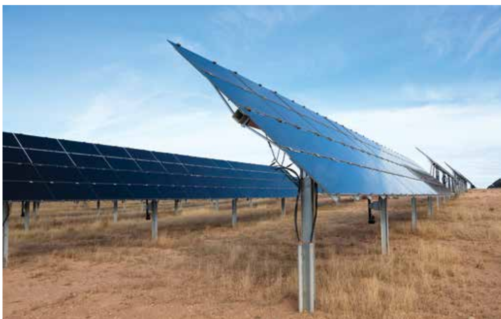
Credit: First Solar
