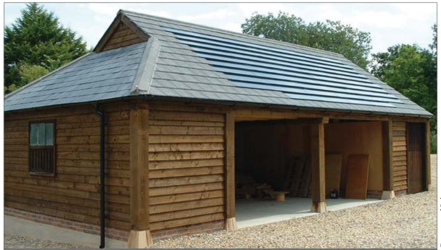
Figure 2. C21e solar electric roof tiles on a building in Sturges Farm, southwest England.
