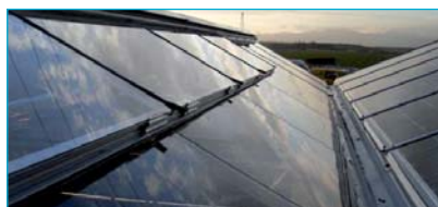
Uni Land installation.
