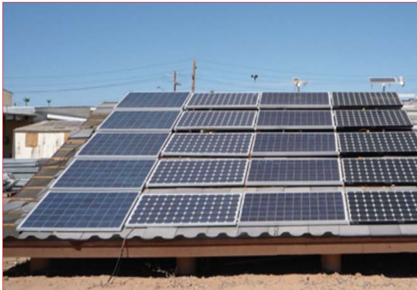
Figure 4. Simulated rooftop structure in the testing yard (front view, bottom row = 0-in. air gap; top row = 4-in. air gap).
