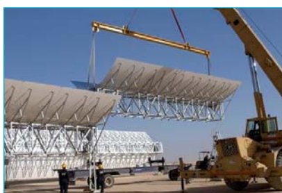
Solar Millennium trough installation.
