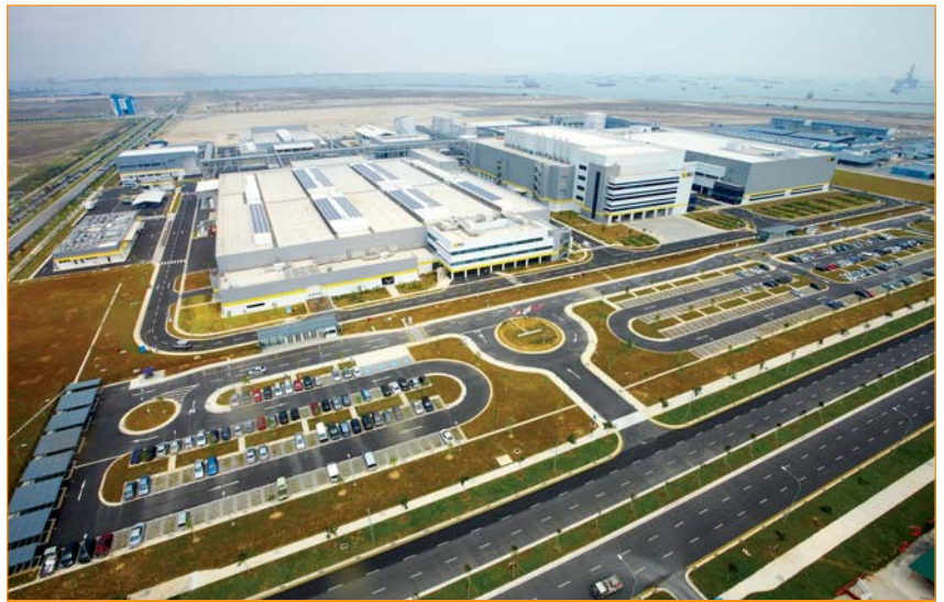
REC Singapore's new integrated PV plant.
