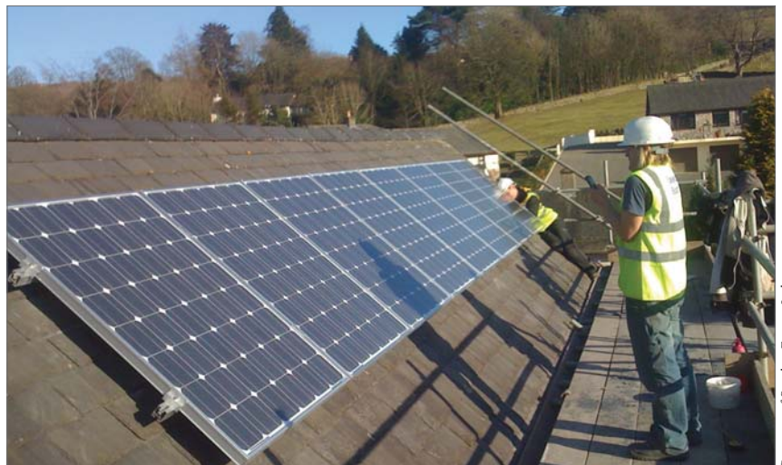
Figure 3. Integrated solar PV on a new build domestic home in south Scotland.
