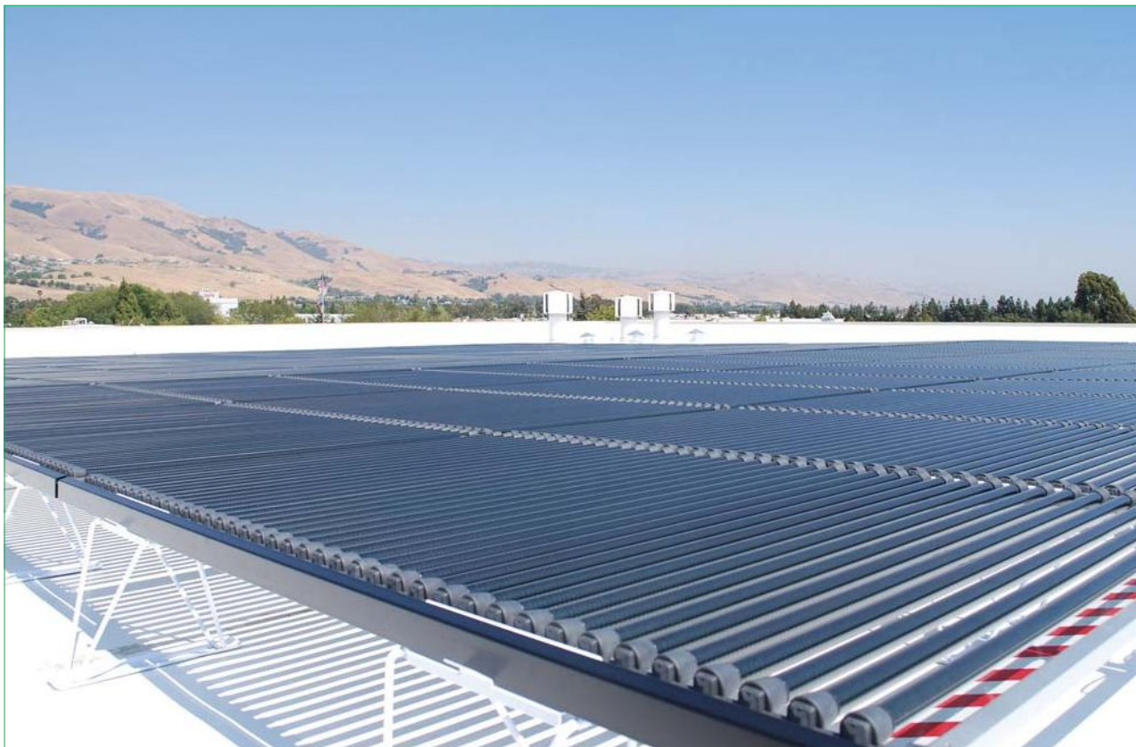
Figure 4. Solyndra claims installation of its rooftop PV panels can be done in about one-third the time and one-half the cost of traditional flat-plate module systems.
