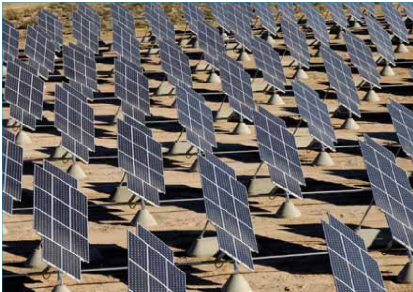
Figure 3. Tilted single-axis trackers optimized for maximum energy production.
