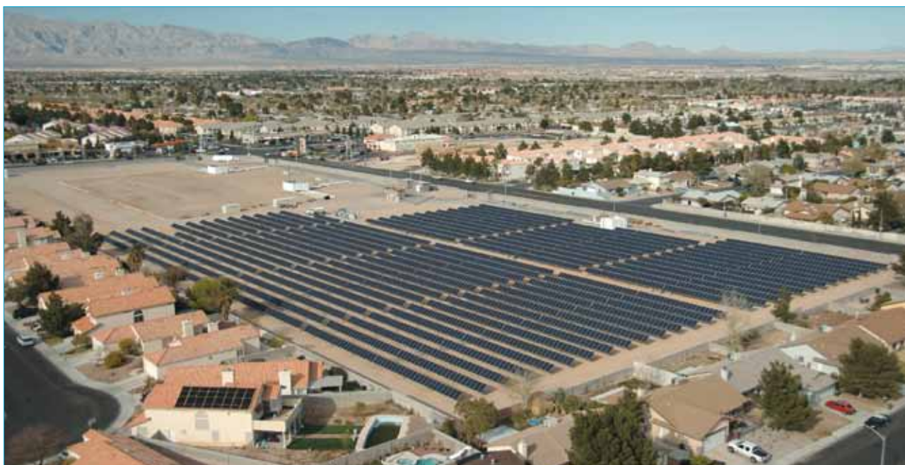
Figure 2. Horizontal single-axis trackers optimized for space-constrained sites.
