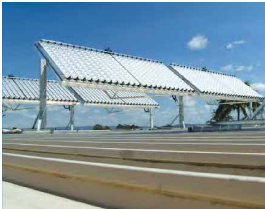
Figure 7. Whitfield Solar's WS:Si24 solar concentrators installed on a residential rooftop in Queensland, Australia.
