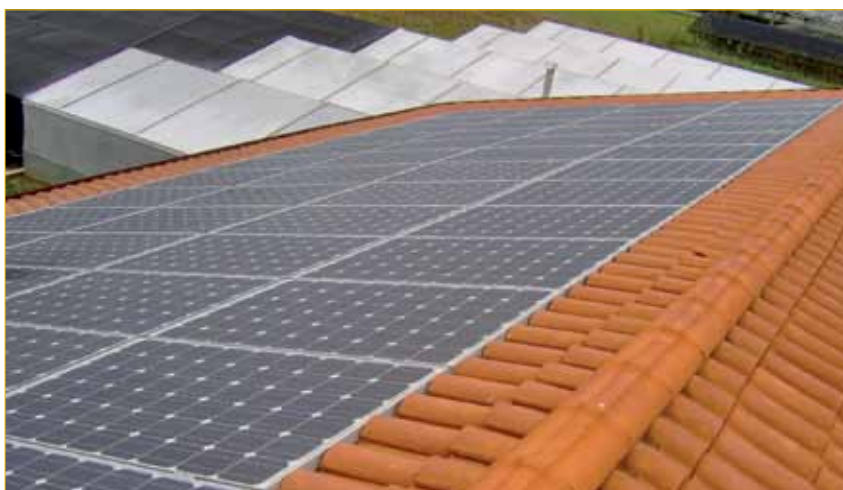
Figure 3. Example of BIPV roof installation.
