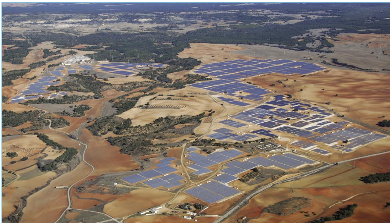
Figure 3. Olmedilla de Alarcon, Cuenca, Spain, a 60MWp installation, was the largest PV power plant constructed in 2008.
