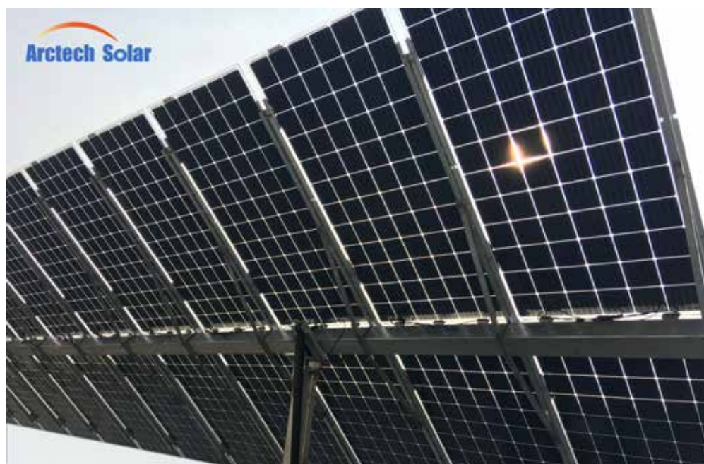
Figure 3. Independent horizontal single-axis tracker from Arctech Solar, designed for bifacial modules [145]. The modules are fixed using aluminium elements at the module edges, overlapping with the long purlins to avoid covering the back of the bifacial modules. Junction boxes at the module edges in such a system, as shown, can be integrated without shading caused by cables.
