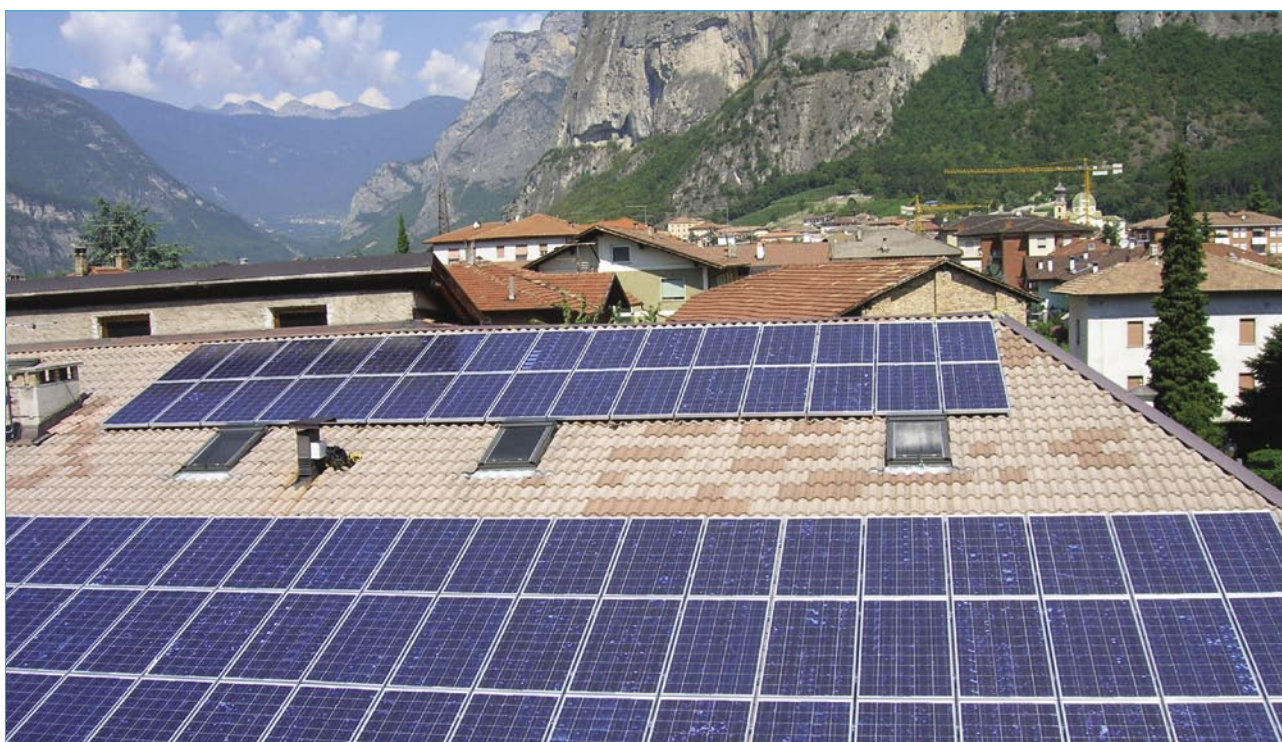
Figure 1. Enerco rooftop installation.
