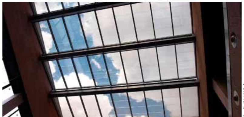
Figure 4. San Antón market (Madrid, Spain) amorphous silicon transparent skylight by ONYX Solar.
