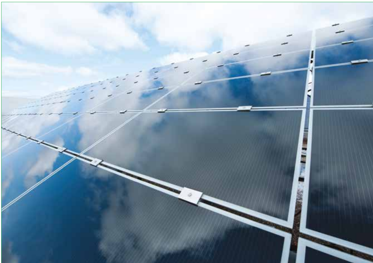
Credit: First Solar
