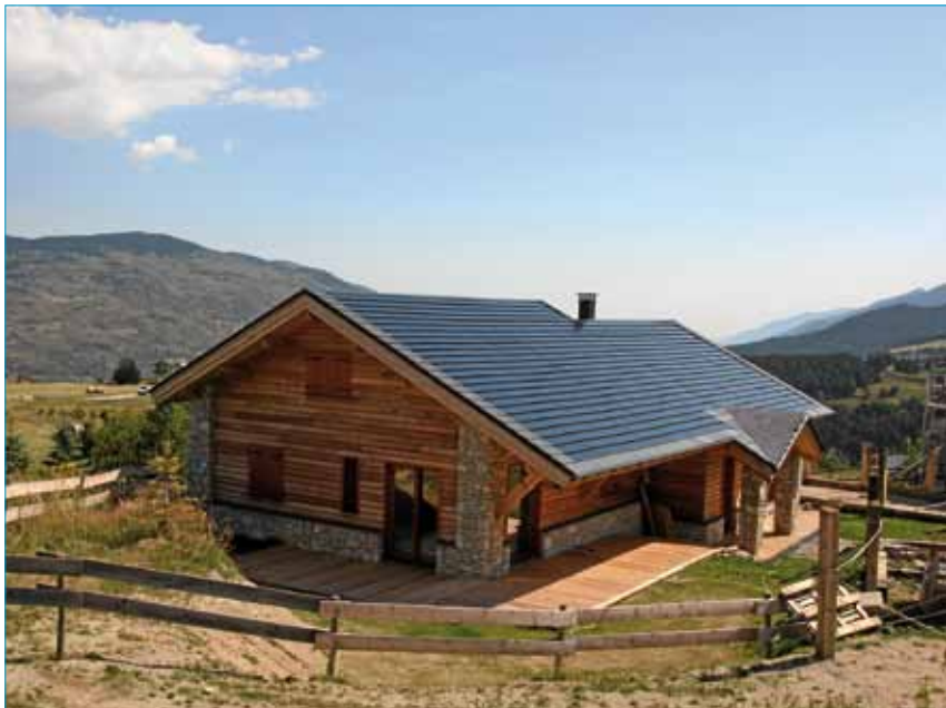
Figure 2. C21e solar electric roof slates in Languedoc-Roussulon, France.
