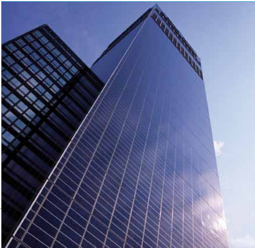
Figure 5. Europe's largest solar façade, the CIS Tower, Manchester, UK.
