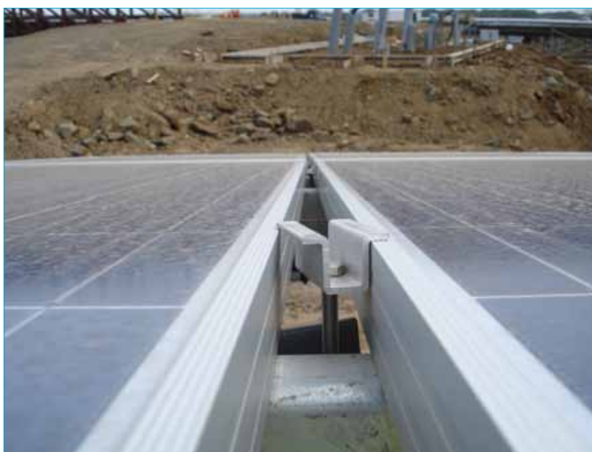
Figure 2. An incorrectly installed omega junction.
