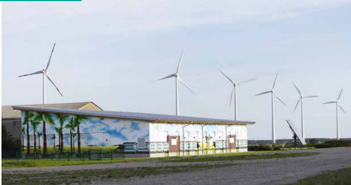
A battery storage park in Feldheim, Germany, co-located with wind turbines. Integrating large volumes of renewables into the grid will be a key long-term driver for storage in Germany
