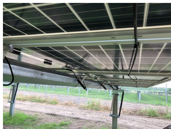
Figure 2. Installation crew familiarity with bifacial modules. To prevent shading of the rear side of the module ensure that crews are properly trained and understand that in addition to the usual wire management considerations the goal is to minimise rear-side shading
