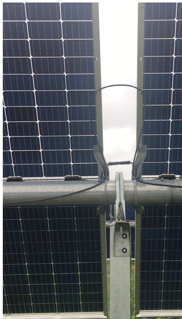
Figure 1. Wiring considerations for bifacial modules: to prevent shading of the rear-side of the module how the DC wire harnesses will travel down the racking structure without shading the rear side of the modules must be considered during the design and procurement stages of the project. Different modules paired with different racking structures require custom approaches
