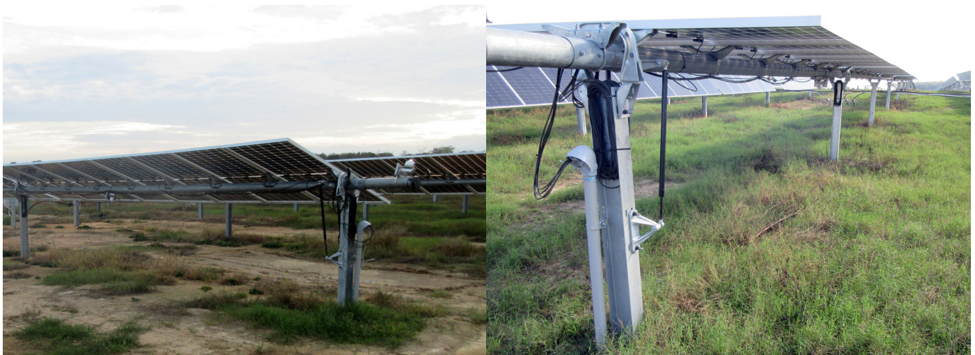
Figure 3. Rear-side irradiance sensor location. Inverter cut-outs, roads, high traffic areas, and natural ground cover variations can result in rear-side POA measurements that are not representative of overall site albedo. Close-ups of the sensors can be found in Figure 4
