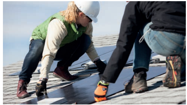
Fraunhofer researchers installing a prototype lightweight PV module in a trial funded by the US Department of Energy.
