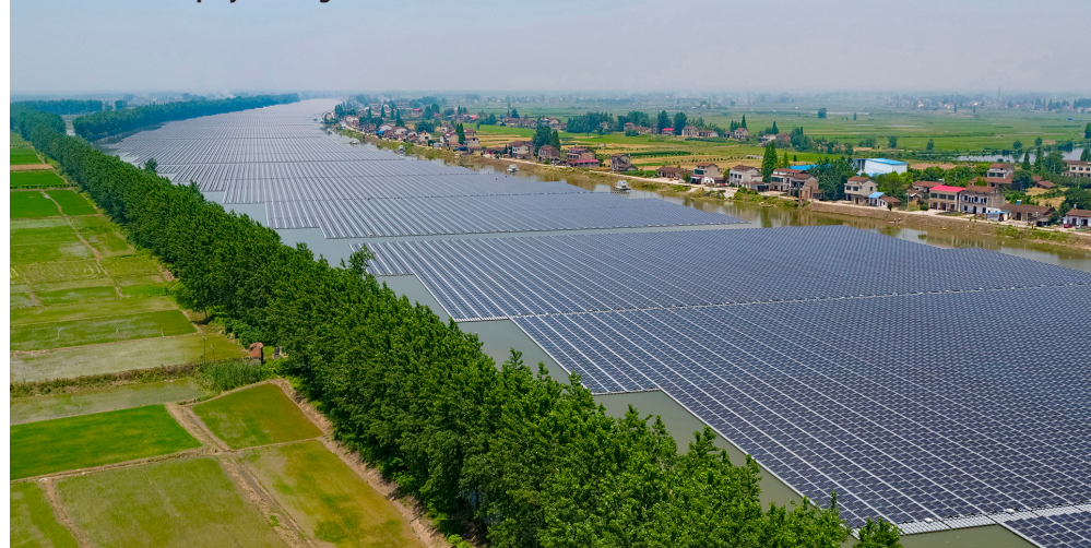
The 100MW FPV project along the Hunan River in China.
