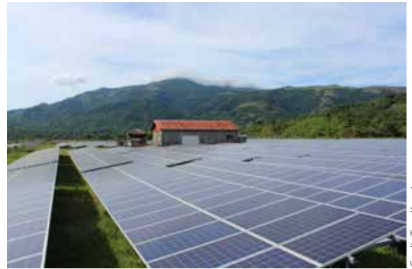
The micro-grid combines 2MW of PV capacity with storage and diesel generators
