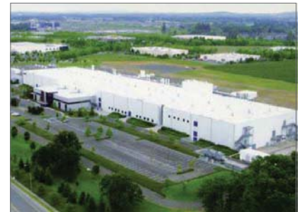
SolarWorld's Hillsboro, Oregon facility.
