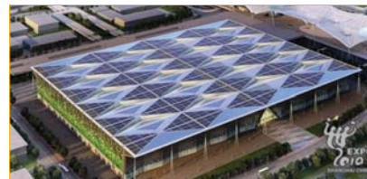
Suntech's BIPV installation, China Pavilion, Shanghai.
