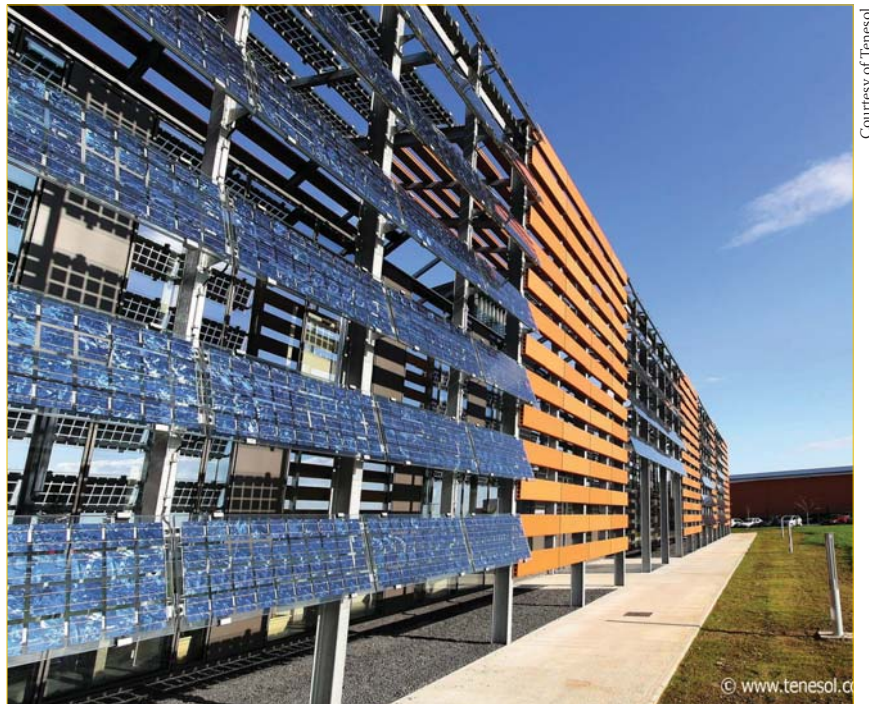
Figure 6. Integrated shading system in a façade.
