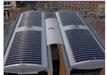
ECD/United Solar Ovonic's solar laminates integrated into a Mario Botta-designed building in Piazza San Lorenzo, Italy.
