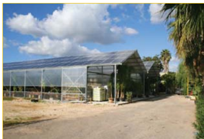
Winsol's 99kWp BIPV greenhouse.
