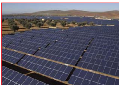
Scheuten Solar's Multisol module array.
