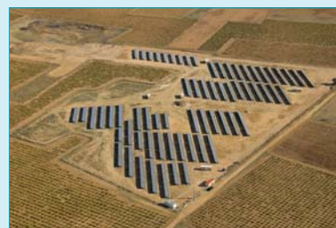
T-Solar power plant at La Seca, Spain.
