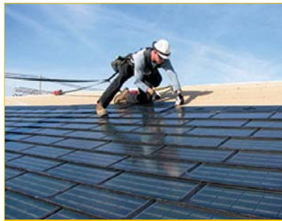
Installation of Dow Chemical's Solar Shingles on a rooftop.
