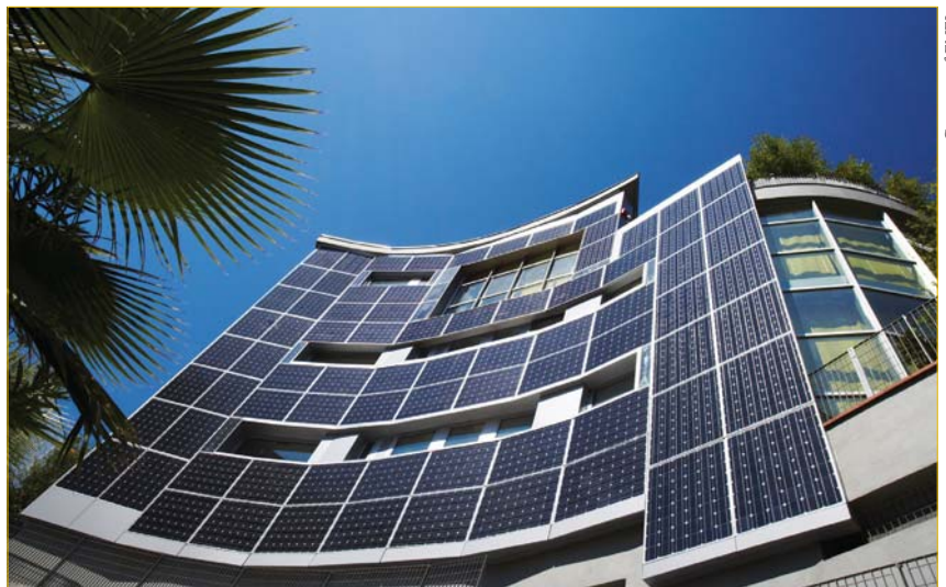
Figure 3. 25KW PV façade for a building's renovation in Cosenza, Italy.
