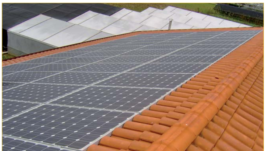
Figure 3. Example of BIPV roof installation.
