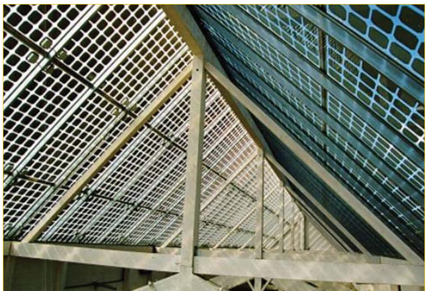
Custom BIPV skylight using AES's BIPV module products.
