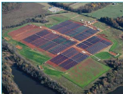
SunEdison's 16MW solar farm in Davidson County, N.C.
