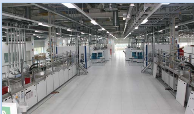
Inside Roth & Rau's production facility.
