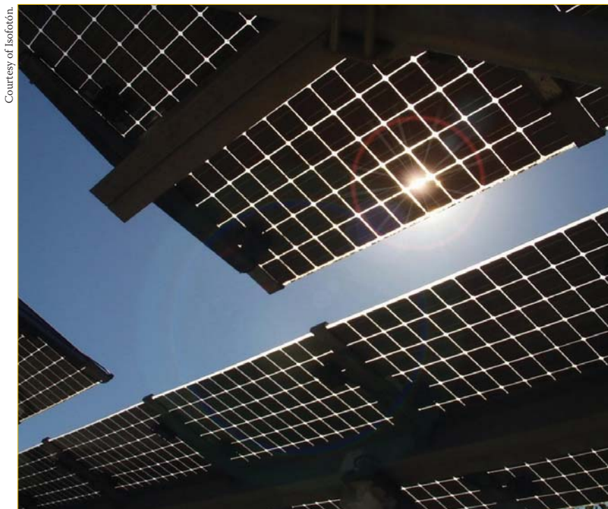
Figure 5. PV pergola acting as a skylight in Spain.
