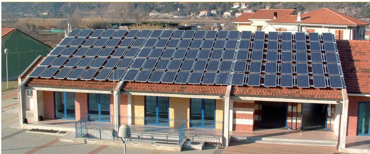
Figure 4. Example of a PV roof installation where the modules exceed the upper line of the roof tiles.
