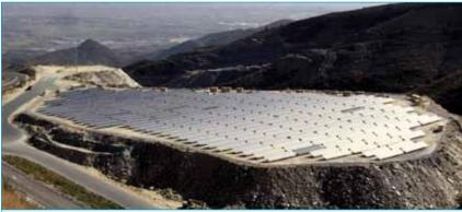
Location: Almería, Spain Nominal power: Phase 1: 2.1MWp; Phase 2: 1.1MWp Free-standing Ground area: Approx. 50,000m<sup>2</sup> Solar modules: Approx. 8,000 units Electricity production: Approx. 2,600,000kWh per annum Completion date: September 2008 Involvement: Concept, Detailed Engineering, Project Finance, Licensing, Negotiations with
