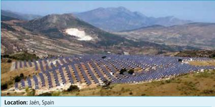
Nominal power: 2.1MWp Trackers: 906 Ground area: Approx. 150,000m<sup>2</sup> Solar modules: Approx. 10,600 units Electricity production: Approx. 4,000,000kWh per annum Completion date: July 2008 Involvement: Concept, Detailed Engineering, Project Finance, Licensing, Negotiations with Public Administrations, Supply Chain, EPC, Optimization, 0&M.
