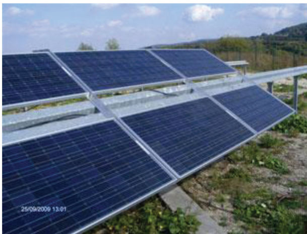
Figure 6. Commercial open-field installation in Saxony, Germany: 8 months with a 20% (0.2) reflectance ground albedo and 12 months with a 50% (0.5) reflectance ground albedo. Results: 17% bifaciality gain over the best module in the field and more than 60% gain in snowy conditions. (The bifacial system kept collecting solar energy through the back side even when the front side was covered with snow, in contrast to all the other systems, which stopped yielding power in these conditions.) The respective cell equivalent efficiency values are 21.7% and 29.6% [13].
