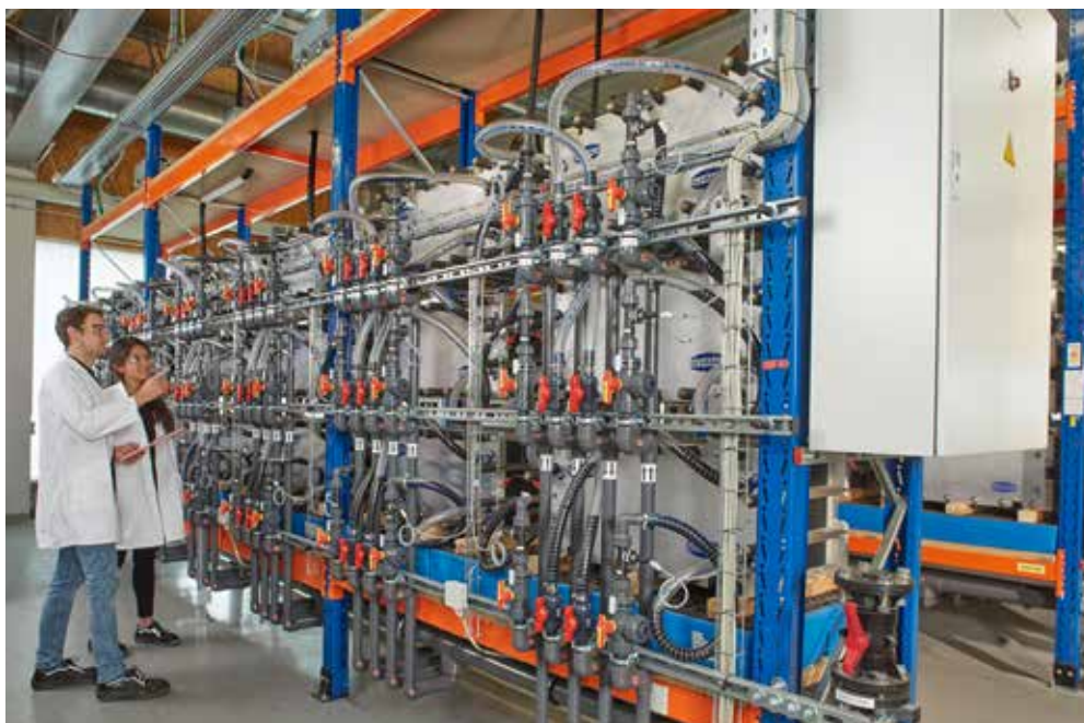
Stacks of a 2MW/20MWh vanadium redox flow battery at Fraunhofer ICT
