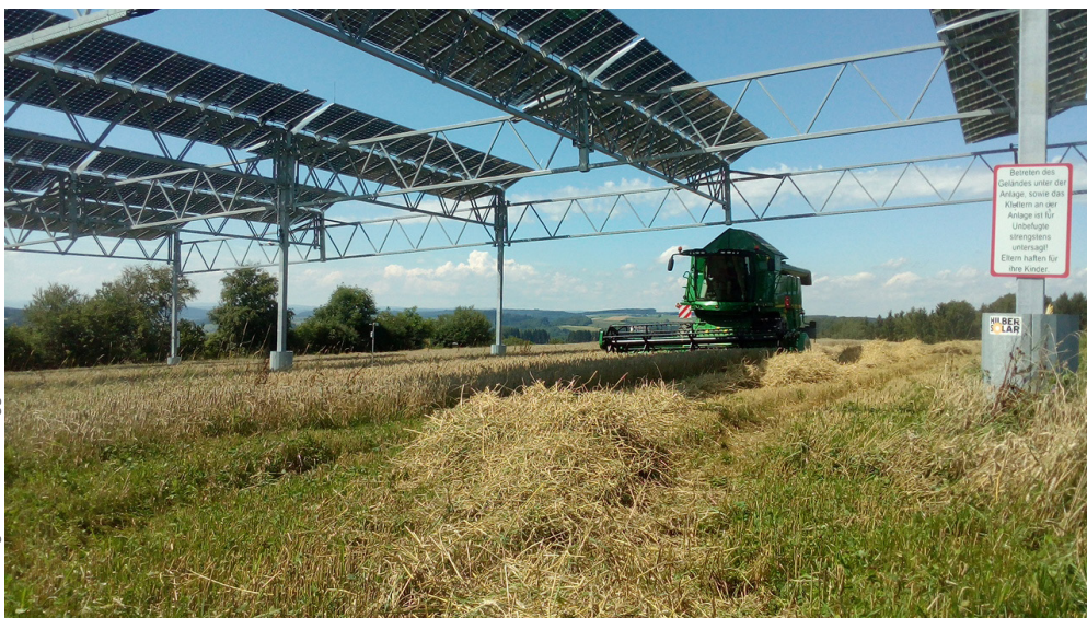
Using agricultural vehicles under an APV system is not a problem. In the future, these could be e-vehicles
