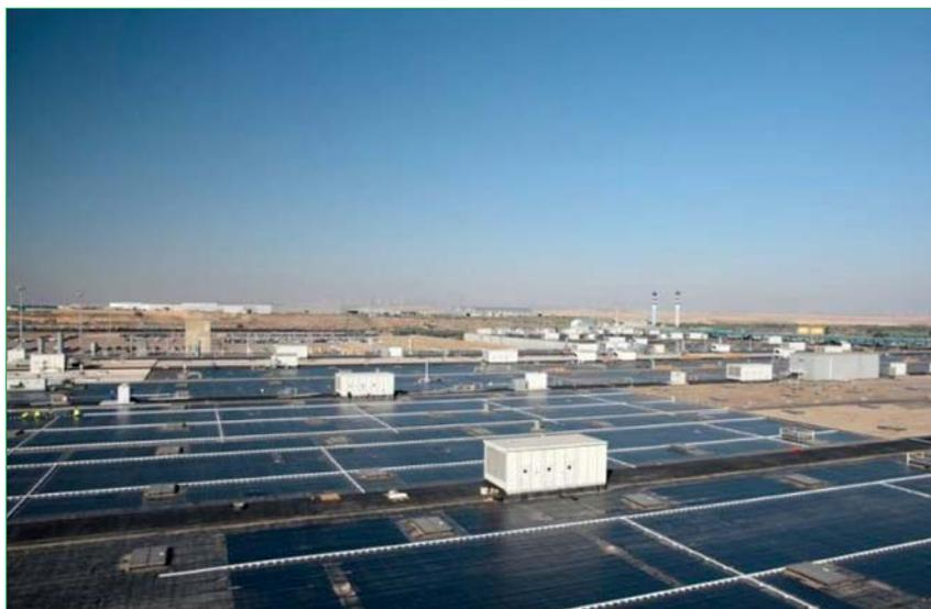
Figure 1. World's largest rooftop system (11.8MW) in Zaragoza, Spain. The system uses flexible thin-film silicon PV laminates.
