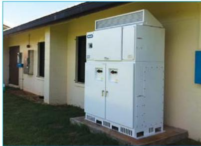
**Advanced Energy's Solaron 500kW PV inverters achieve 98% efficiency**
