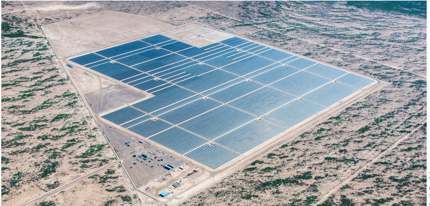
Credit: First Solar
