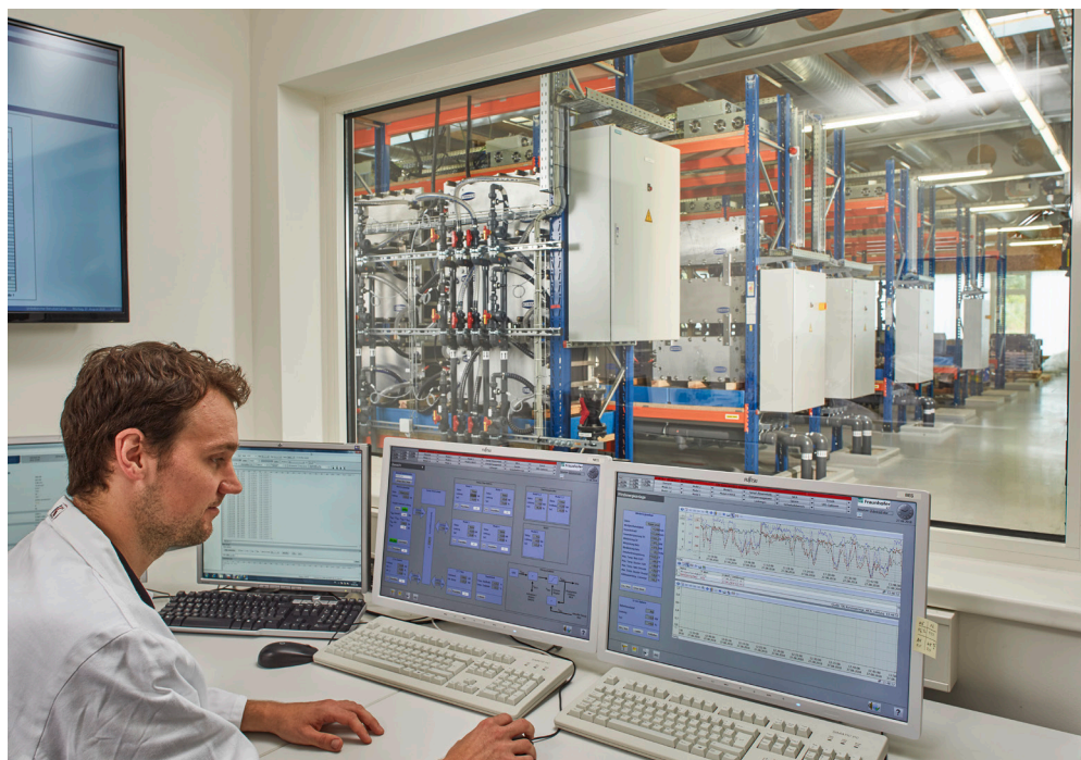
Figure 6. Control room of a 2 MW/20 MWh vanadium redox flow battery at Fraunhofer ICT
