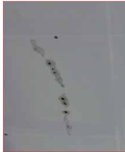
Figure 5. Affected cell crack with smouldering and arcing along the defect.
