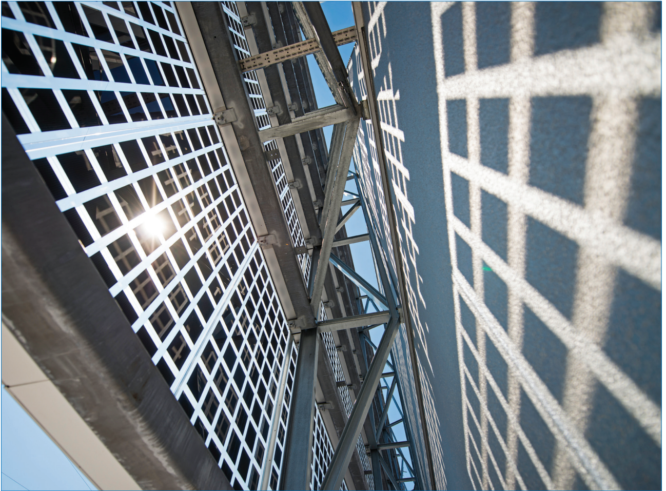
Figure 3. Semi-transparent facade of the renovated CSEM building in Neuchâtel, Switzerland, which comprises bifacial silicon heterojunction solar cells that are interconnected using SmartWire Contacting Technology [17].
