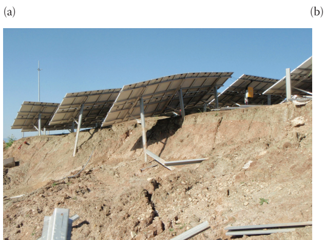
Figure 9. Damage to a PV system: (a) from ground subsidence; (b) from fire.
